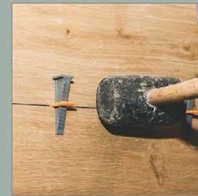
Remove Wedges Ones It Dry
