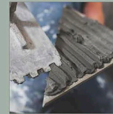
Cement Laying On Tile
