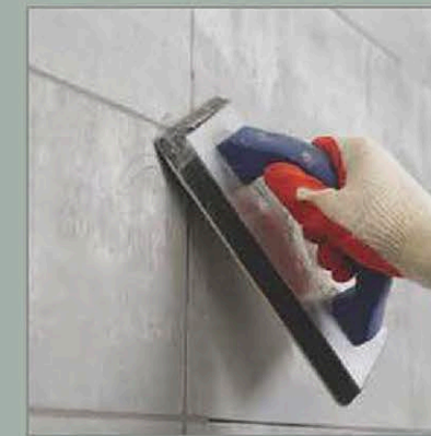
Joint Grouting
