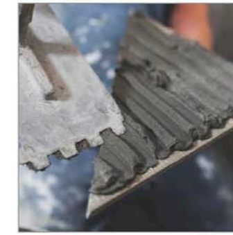
Cement Laying On Tile
