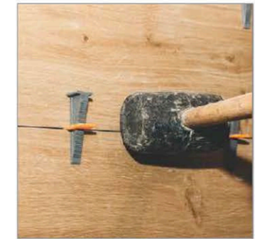
Remove Wedges Ones It Dry
