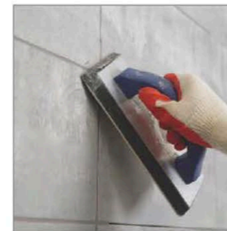
Joint Grouting
