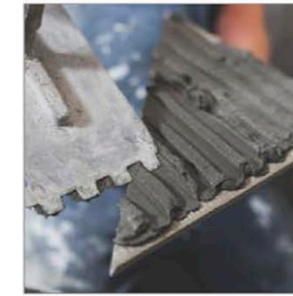
Cement Laying On Tile
