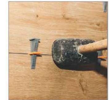
Remove Wedges Ones It Dry
