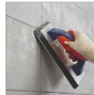
Joint Grouting
