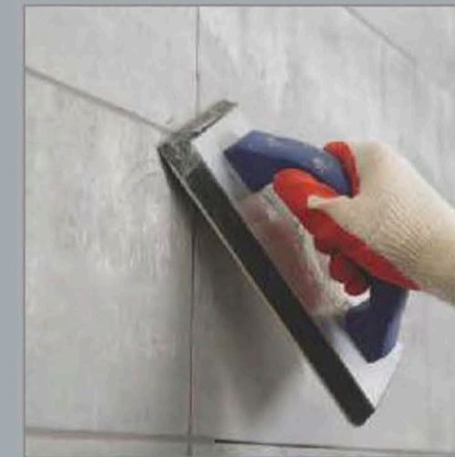
Joint Grouting
