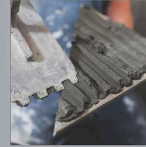
Cement Laying On Tile
