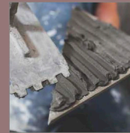
Cement Laying On Tile
