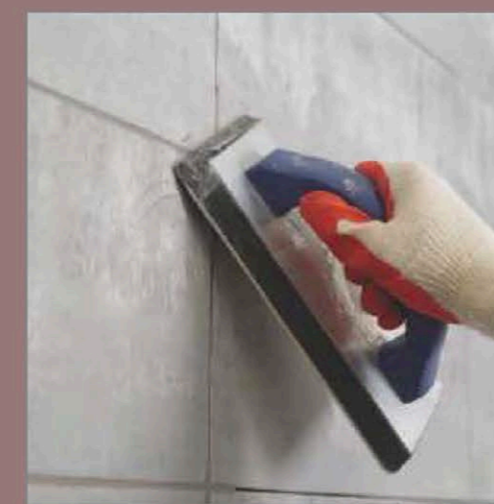
Joint Grouting
