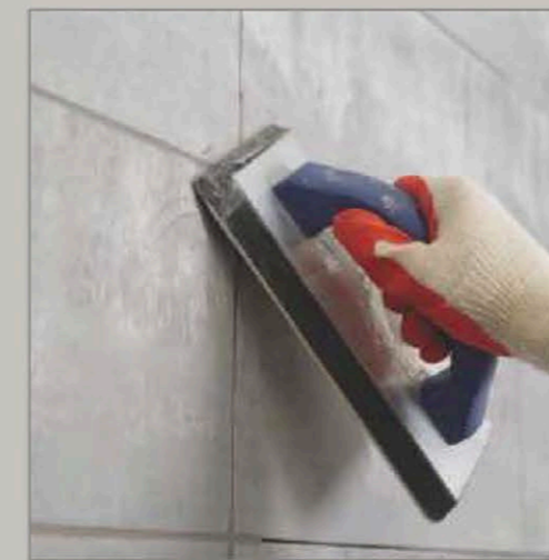
Joint Grouting
