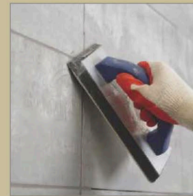
Joint Grouting
