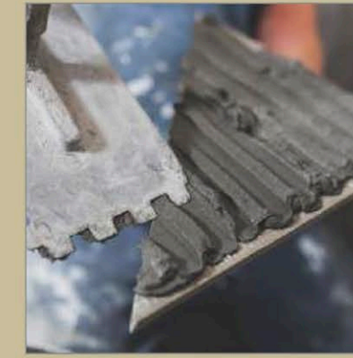
Cement Laying On Tile
