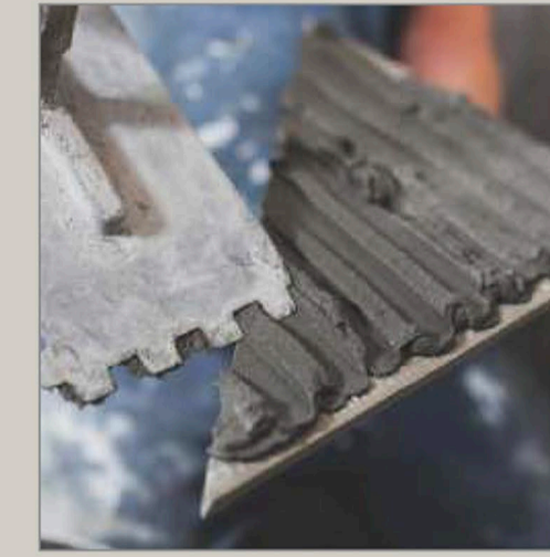
Cement Laying On Tile
