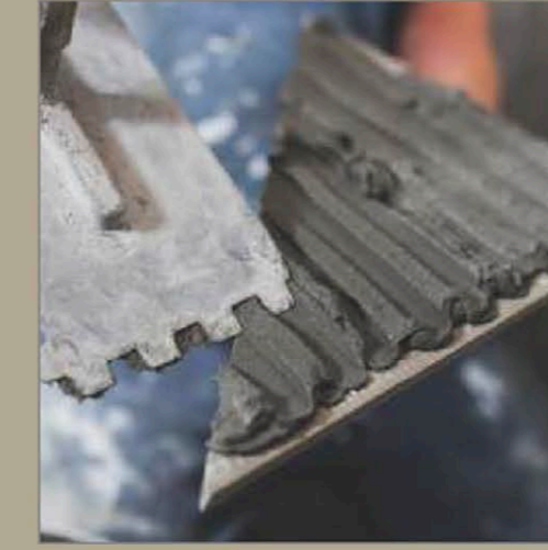
Cement Laying On Tile
